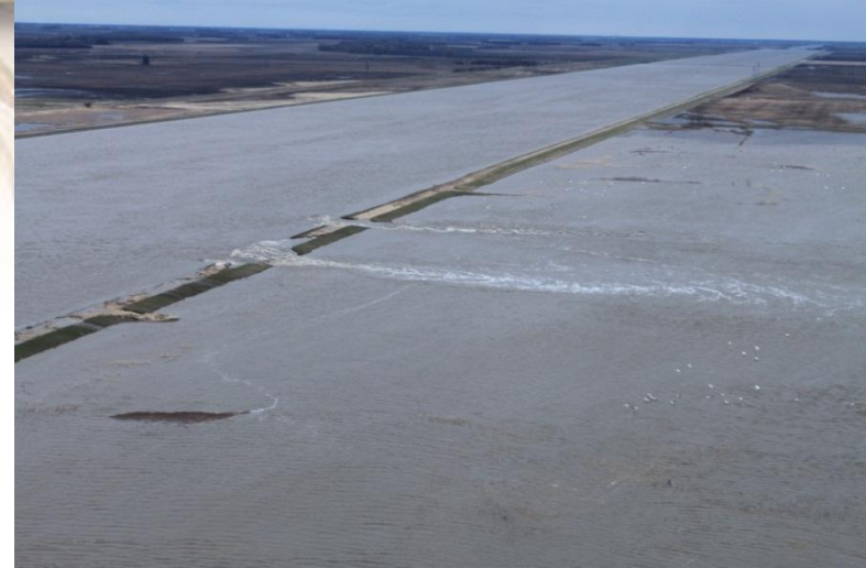
2011 Assiniboine River Flood - Breach in the Assiniboine Diversion Dike (above); Floodwaters surround a farm operation and rural homes west of Winnipeg (below). Costs from the 2011 Manitoba Flood have exceeded $1 billion with over $320 million going to the agriculture sector in Agri-Risk and Recovery Programs.
